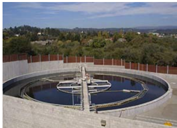
Waste Water Treatment Plants
